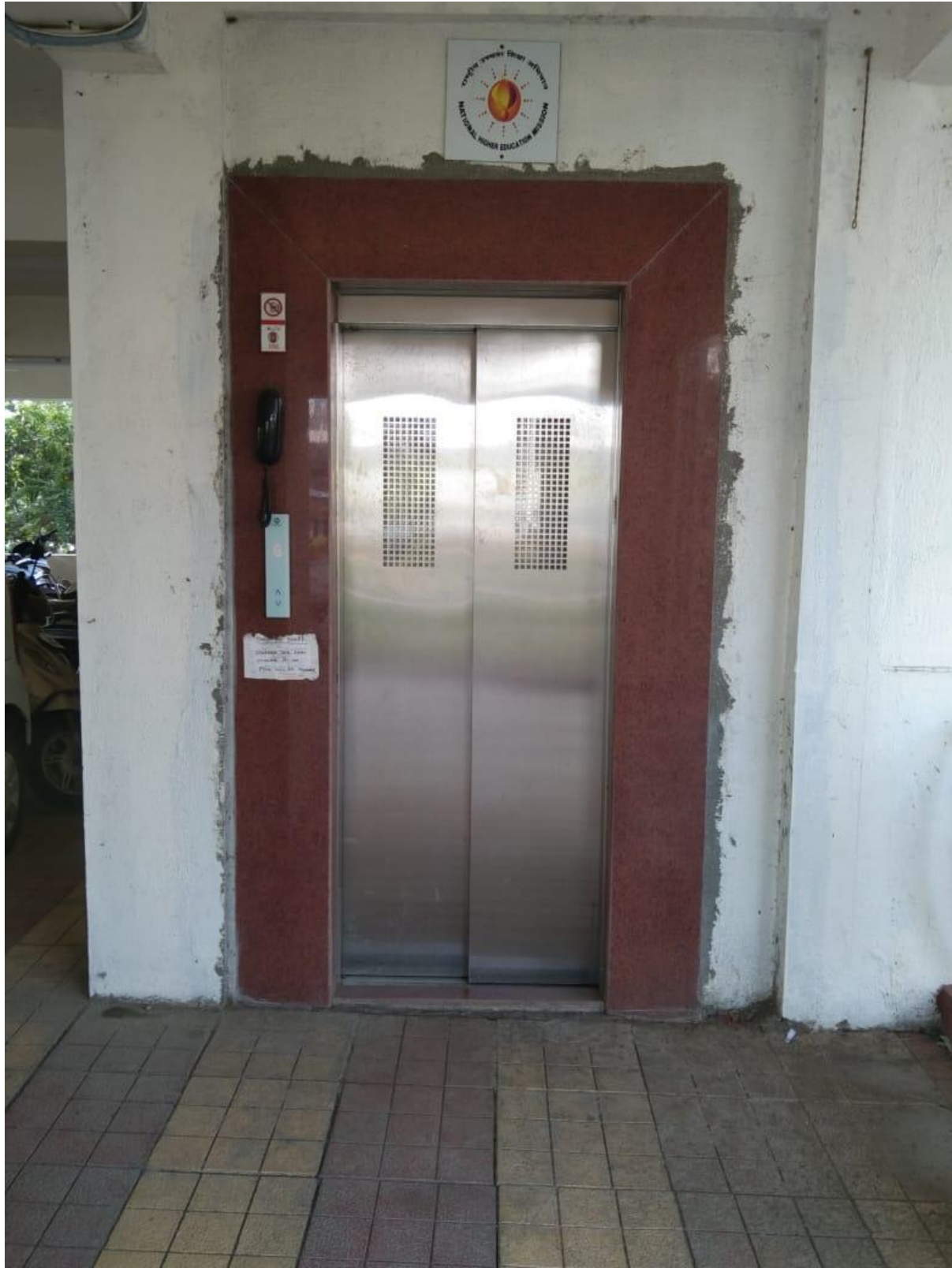
Creation of the Lift Facility in the Gymkhana Building
